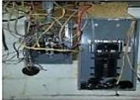
Damaged insulation
