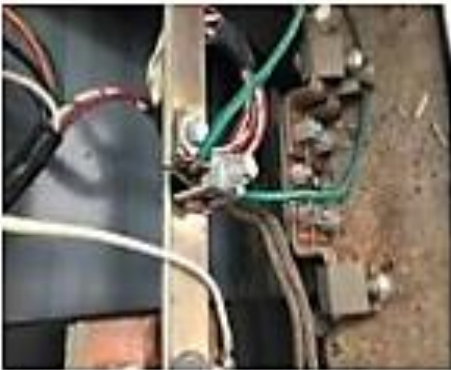
Improper grounding
