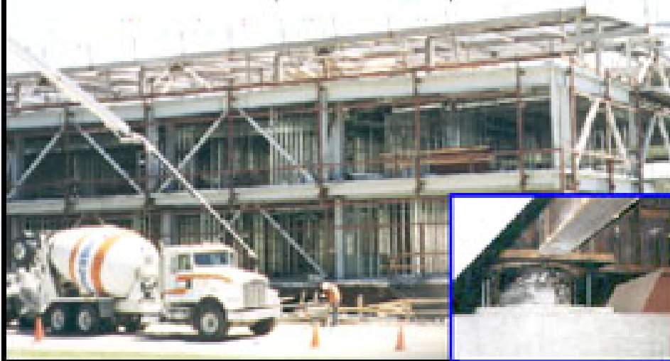
Construction of hospital in earthquake zone
