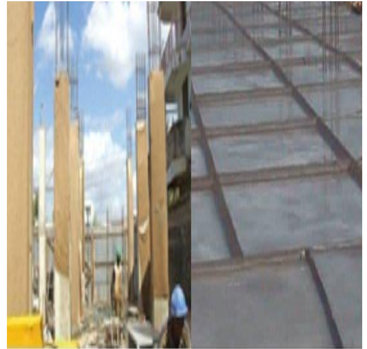
Curing of Vertical surfaces Curing of Horizontal surfaces
