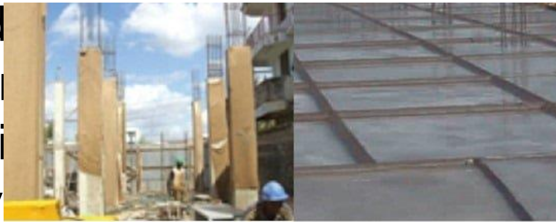
Curing of Vertical surfaces Curing of Horizontal surfaces
