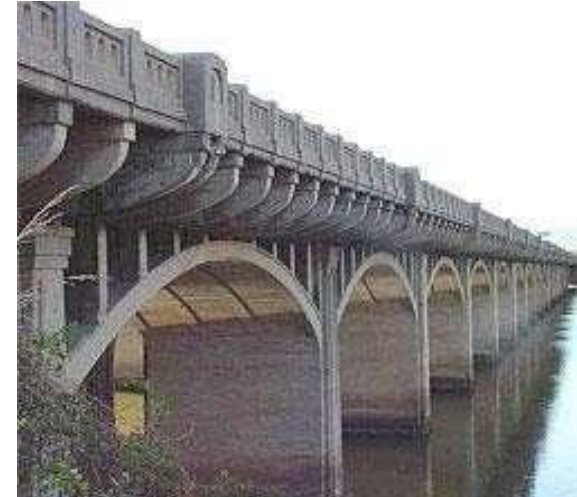
Monolithic Concrete Arch
