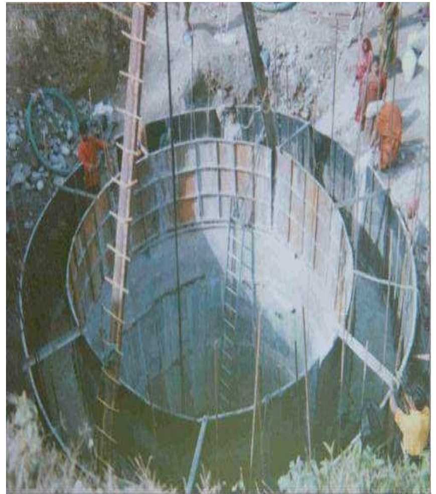
SHUTTERING WORK IN PROGRESS WELL FOUNDATION OF SIMBLE Br AT KM 18.044 ON SIMBLE Br JAMMU-AKHNOOR ROAD
