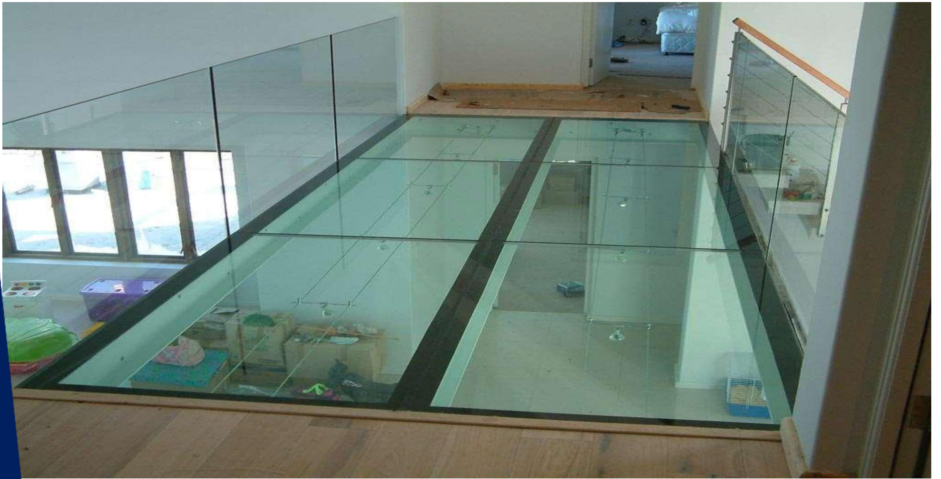
Figure 1: A glass floor panel installed in a room, showing the reflection of the room below.
