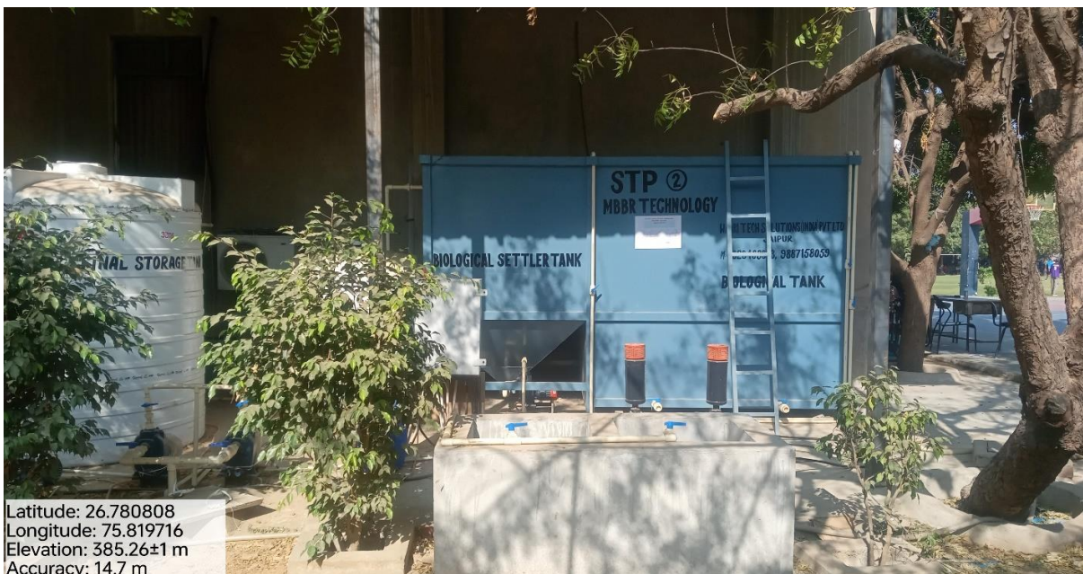
Sewage Treatment Plant
