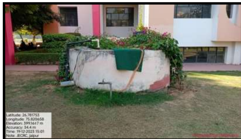
Rain Water Harvesting Tank
