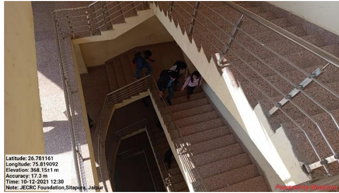
Good daylight and Ventilation in classrooms Main staircase which receives daylight
