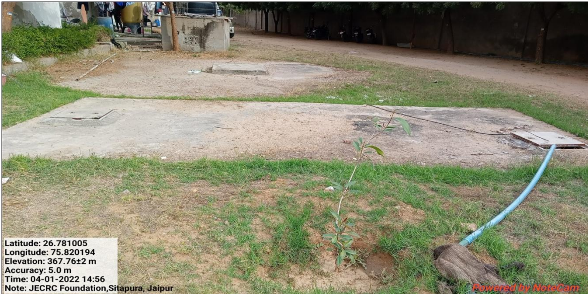
Septic Tank (Liquid Waste Management)
